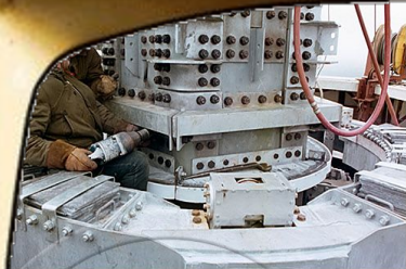
CANRON 'Bolting Gang' Tightening 1 of 30,000 Bolts
