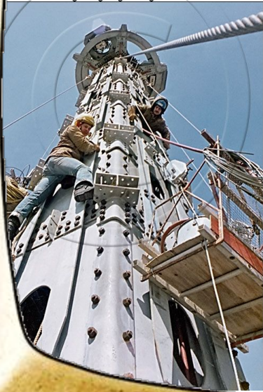
ANRON 'Bolting Gang' Tightening 1 of 30,000 Bolts
