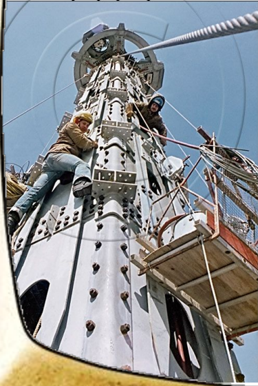
CANRON 'Bolting Gang' Tightening 1 of 30,000 Bolts
