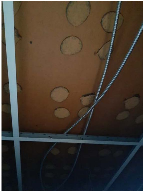
Photograph No. 15 – Mastic was sampled above the drop ceiling in room 215 and does not contain asbestos.
