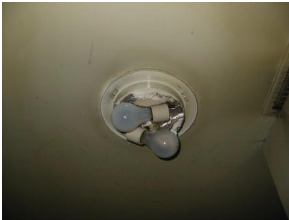
Paper heat shield on incandescent fixture
