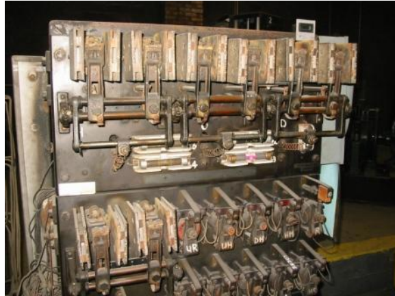
Transite Blocks in Elevator Switchgear
