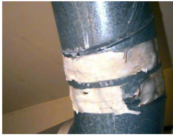
Paper on seams of duct
