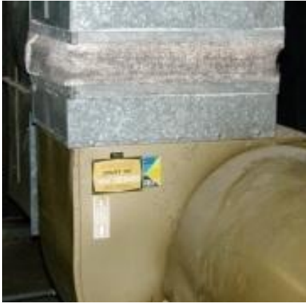
Textile Vibration Damper/Duct Connector
