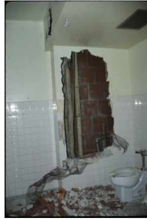
Plaster on speed tile
