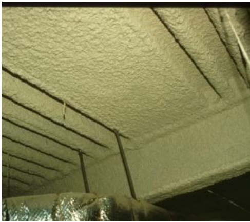
Cementitious sprayed fireproofing
