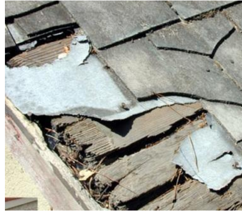
Building paper under roof tiles
