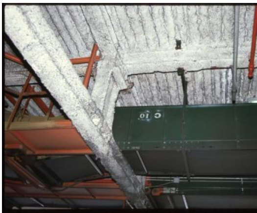
Fibrous sprayed fireproofing
