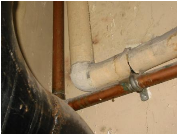
Parging cement on pipe fitting
