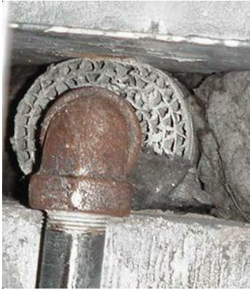
Aircell insulation (corrugated paper)
