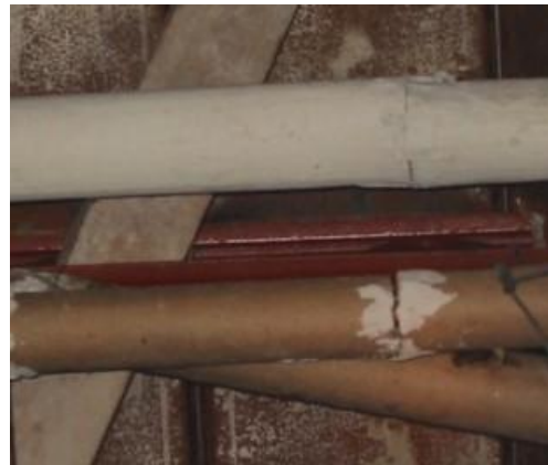
Parging cement on sweatwrap and Aircell
