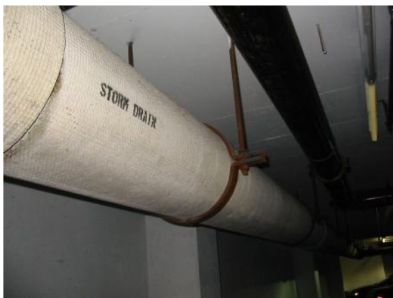
Transite Drain Pipe
