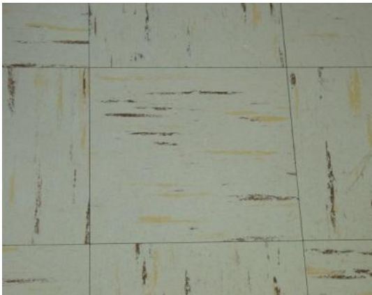
Vinyl asbestos tile
