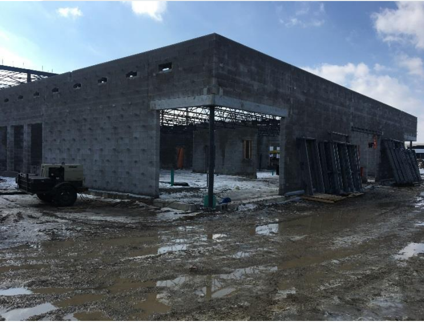
Block wall, structural steel construction at childcare
