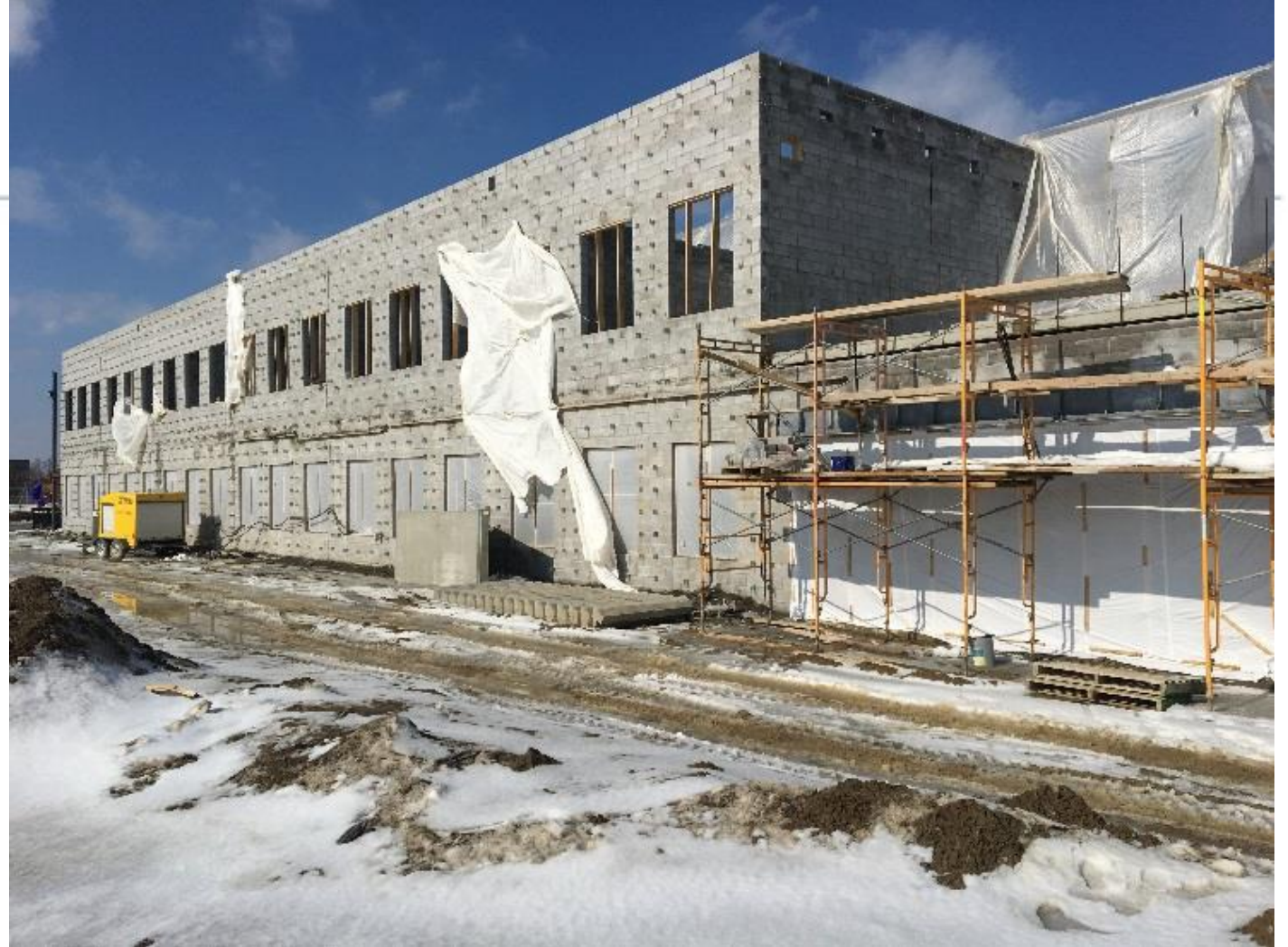
Block wall and structural steel construction of second floor
