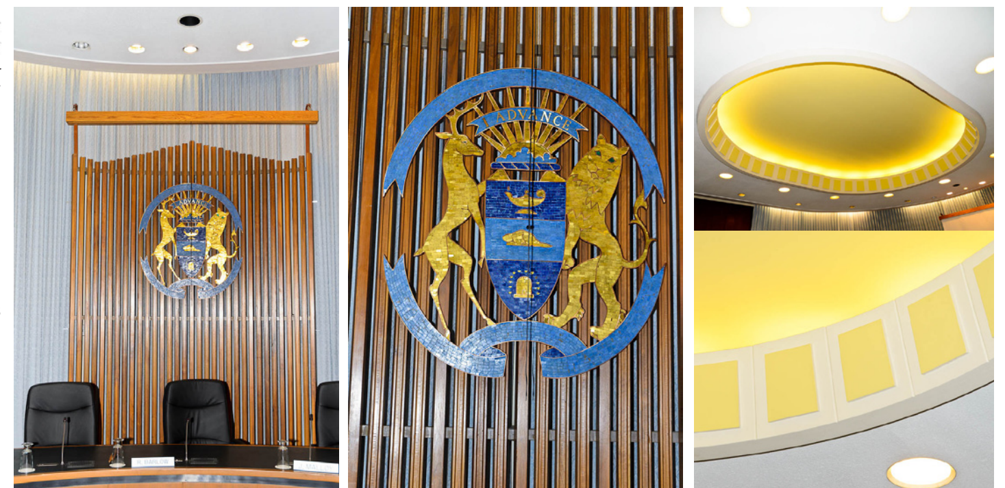
Board room details clockwise from left: walnut screen with Board crest; detail of Board crest; acoustic plaster ceiling; detail of acoustic plaster
