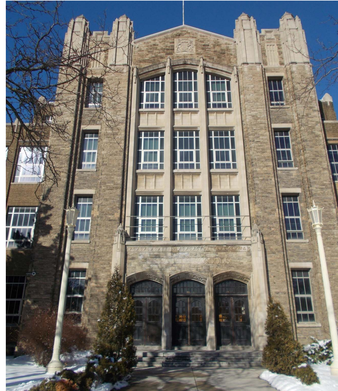
Image 1 – School Main Entry
