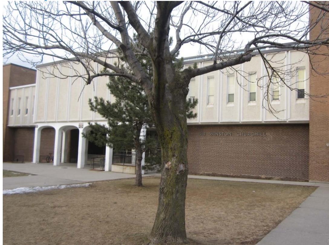
Image 1 – School Main Entry
