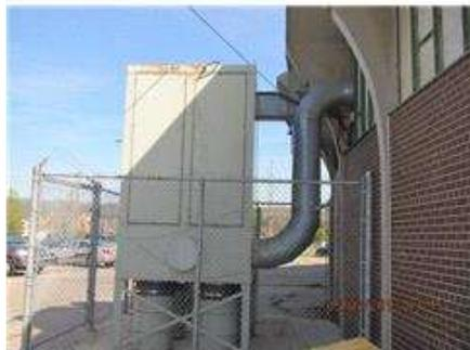
May 2013 - Minor Corrosion of Dust Collector
