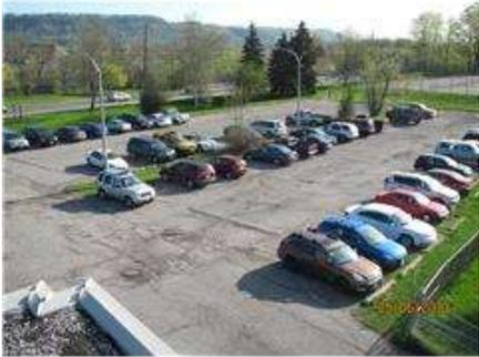
May 2013- Alligator cracking and potholes on the surface of parking lot.
