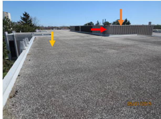
Photograph 2 – S/E view from north-west corner of Area B1 Orange arrow – Area A1, Blue arrow – Area B1 Red arrows – masonry failure requires remedial work
