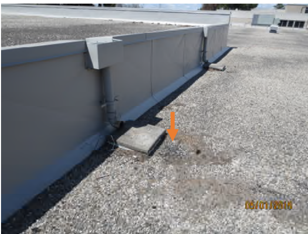
Photograph 23 – View at east perimeter Area F1 Orange arrow – water discharge from Area F1 washing out gravel on Area E2
