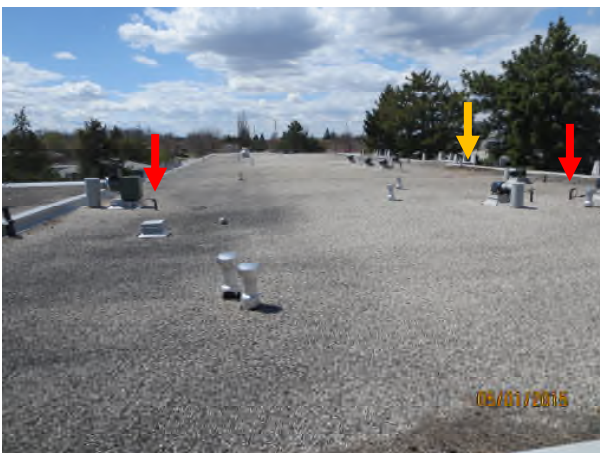
Photograph 11 – West view of Area D2 Yellow arrow – vegetation Red arrows – conduit sleeves not sealed or mastic cracked
