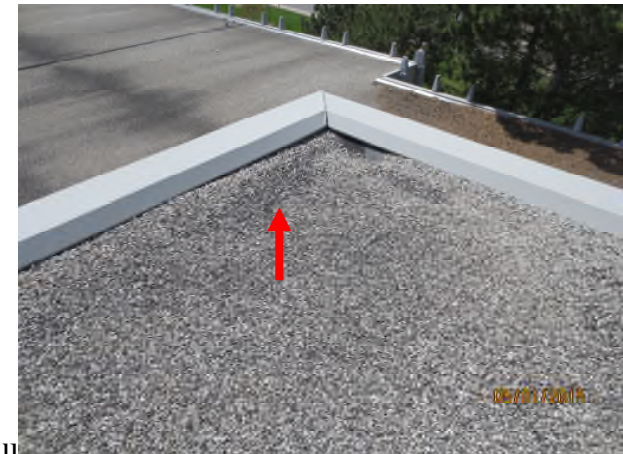
Photograph 4 – S-W corner on Area A1 Red arrow – view of gravel scoured corner exposing bitumen/felt
