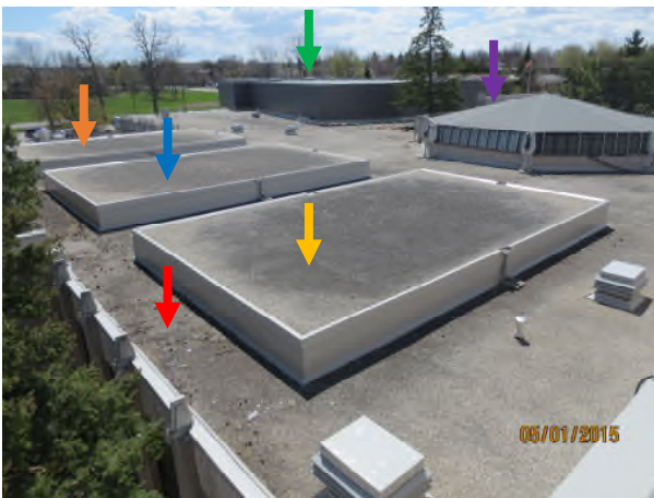
Photograph 27 – South-west view from Area D2 Orange arrow – Area H1, Blue arrow – Area H2 Yellow arrow – Area H3, Green arrow – Area G1 Purple arrow – Area K1, membrane weathered Red arrow – extensive vegetation/debris
