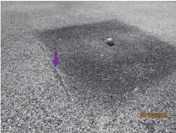
Photograph 7 – Close-up view of drain area in Photo# 6 from Area C3 Purple arrow - exposed membrane felt at transition to sump
