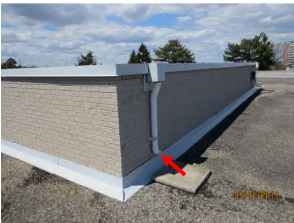
Photograph 17 – N/W view of Area D4 Red arrow – damaged downspout
