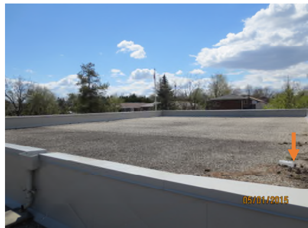
Photograph 24 – S/W view of Area F1 Roof system in fair condition Orange arrow – vegetation/debris to bed removed
