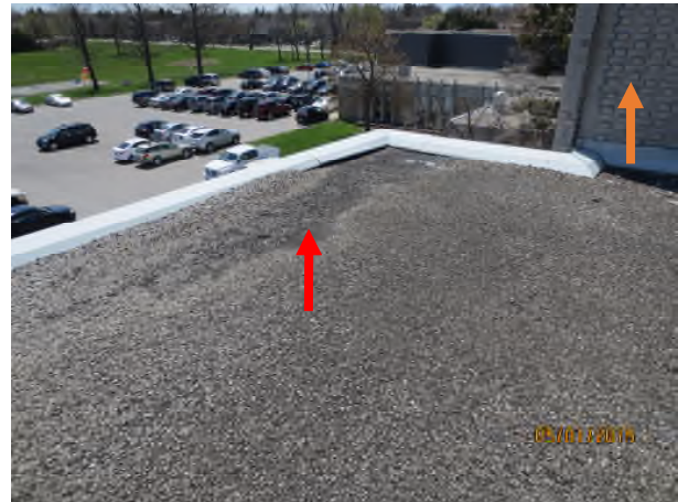
Photograph 14 – View at S/W corner of Area D1 Red arrow – excessive gravel scouring and exposed bituminous felt Orange arrow – masonry chimney required repairs
