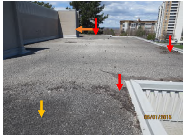
Photograph 20 – North view of Area J1 Red arrow – minor vegetation/debris Yellow arrow – evidence of water ponding
