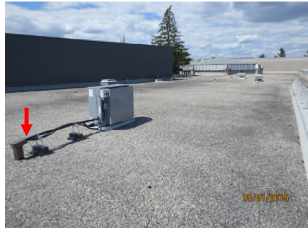
Photograph 26 – N/W view Area E2, east section Red arrow – conduit penetration not sealed
