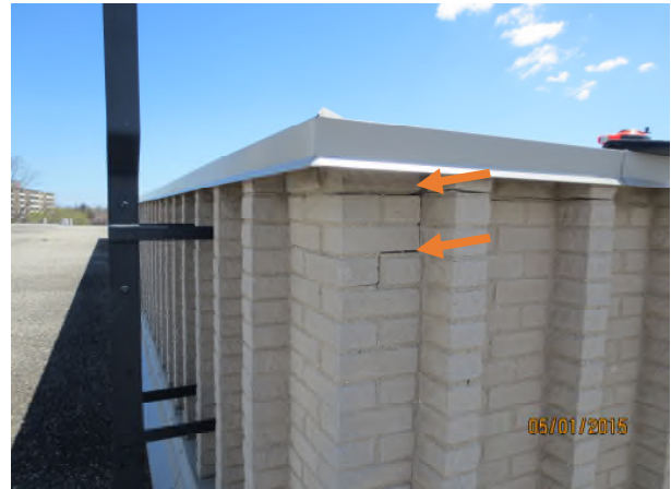
Photograph 32 – North-west corner of Area A1 Orange arrows - cracked mortar joints and dislodged masonry units
