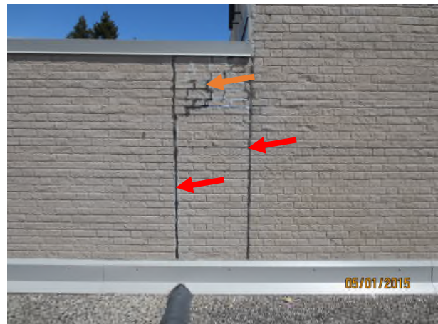
Photograph 34 – View of failed joint on east wall between Area E1 & E2 Orange arrows - cracked mortar joints Red arrows – failed sealant joints
