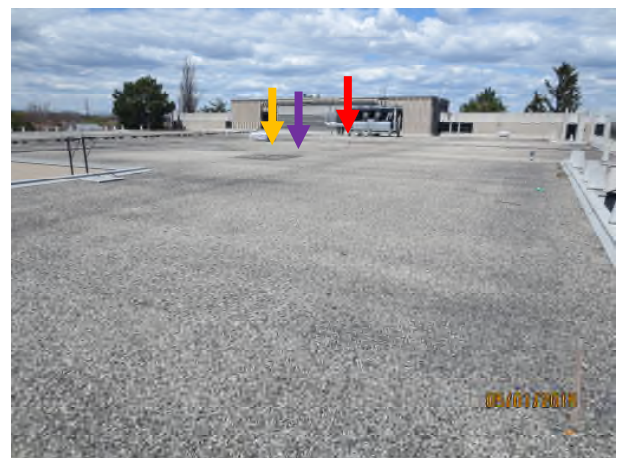
Photograph 6 – N/W view from Area C3 Yellow arrow – drain area with debris Purple arrow – exposed membrane felt Red arrow – damaged vent sleeves
