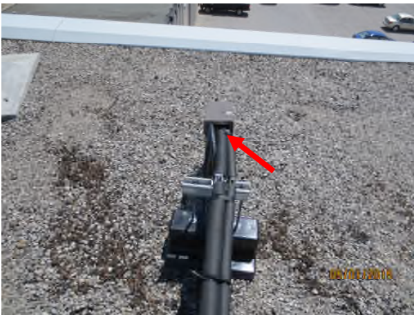
Photograph 15 – View at south side of Area D1 Red arrow – conduit sleeve open to moisture infiltration
