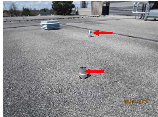
Photograph 8 – View at north side Area C3 Red arrows – damaged vent sleeves
