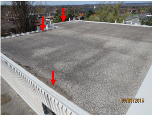
Photograph 3 – N-W view of Area B1 Red arrows – vegetation/debris on roof surface
