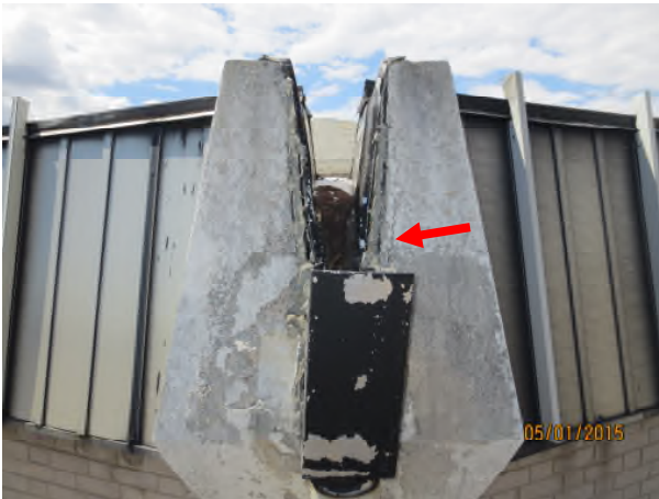
Photograph 31 – View at scuppers locations on Area K1 Red arrow - concrete spalling at several locations and will require repairs
