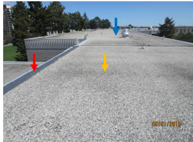
Photograph 10 – East view from area D3 Yellow arrow – Area D3, Blue arrow – Area D2 Red arrow – metal flashing blow-off
