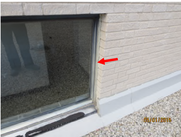
Photograph 35 – Sealant failure at windows above Area E1
