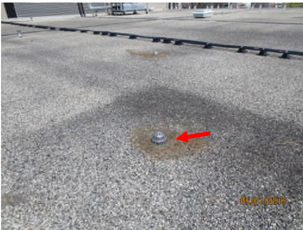
Photograph 33 – View of typical drain clogged with vegetation
