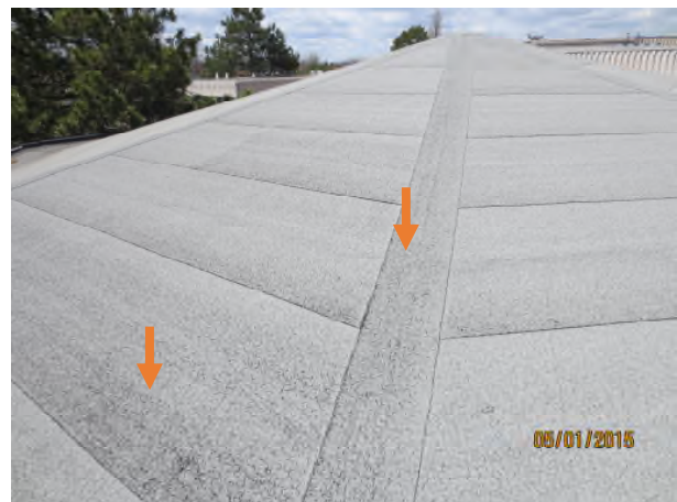
Photograph 30 – N/W view of Area K1 Red arrows – mod. bit. membrane weathered, with 'alligating' n bitumen surface
