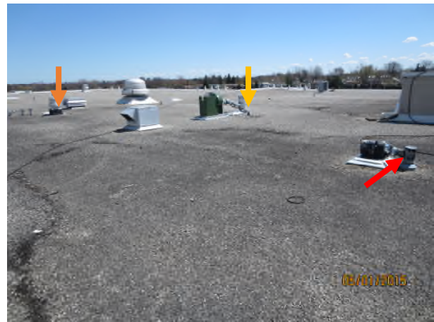
Photograph 16 – S/E view of Area D1 Orange arrow – membrane flashings required repairs at seams Red arrow – abandoned unit Yellow arrow – mastic in pitch-pan failing
