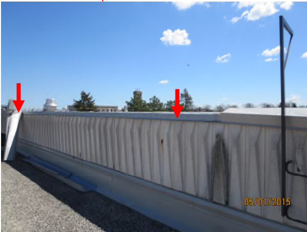
Photograph 9 – View of north perimeter Area D3 Red arrows – metal cap flashing blow-off / damaged/missing
