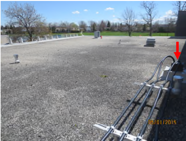
Photograph 25 – S/E view Area E2, east section Red arrow – sealant at conduit penetration failing
