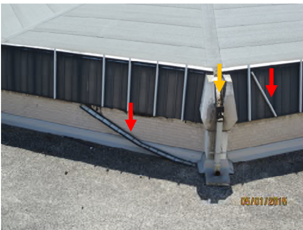
Photograph 29 – View at north side Area K1 Red arrows - damaged soffit, metal cap Yellow arrow – vegetation in scupper
