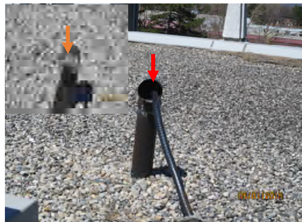
Photograph 12 – Close-up view of typical conduit sleeve on Area D2 Red arrow – no sealant, open to moisture Orange arrow – sealant cracked
