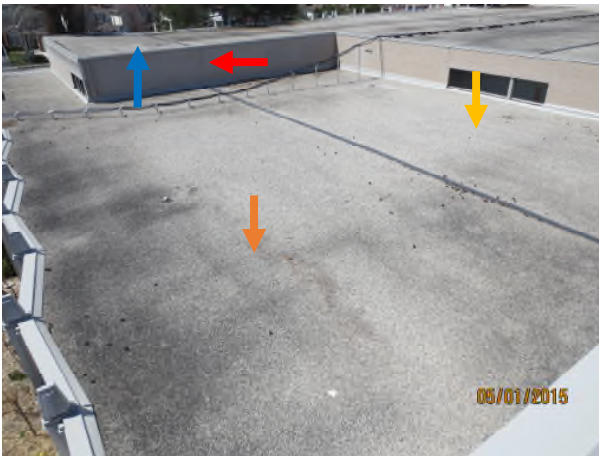
Photograph 21 – N/W view from Area D3 Orange arrow – Area E2, Yellow arrow – Area E1 Red arrow – joint failure, also on east wall Blue arrow – Area C5
