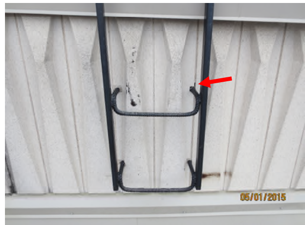
Photograph 36 – Penetration through precast walls not sealed
