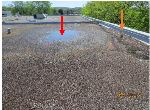
Photograph 14 – South-west corner on Area 501 Red arrow – ponding water on roof surface. Consider new drain at this location when re-roofing Orange arrow – excessive vegetation and 'tree growth'
