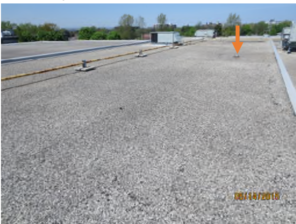
Photograph 33 – North view of Area 701 Orange arrow – minor debris around drain,
