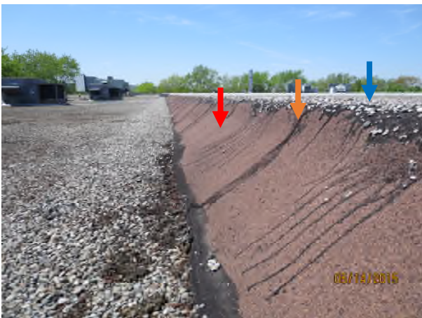
Photograph 23 – Close up view of in Photo#21/22 Orange arrow – open side overlap Red arrow – slippage and blistering along entire joint Blue arrow – no gravel stop on Area 601
