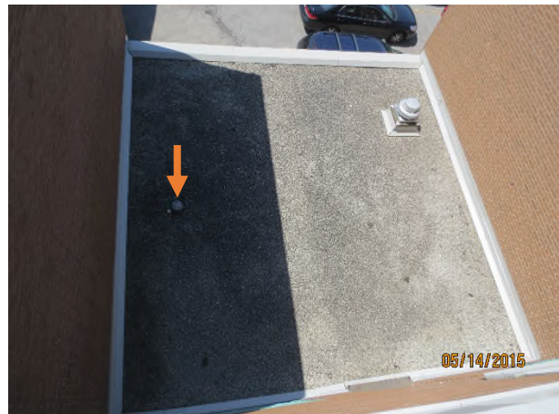
Photograph 26 – West view of Area 202 Orange arrow – debris around drain
