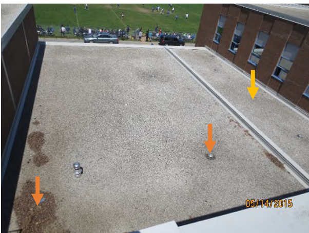
Photograph 29 – N/E view of areas 305(Left) & 306(Right) Orange arrows – debris/vegetation on Area 305 and drain area clogged Yellow arrow – Area 306 – in good condition
