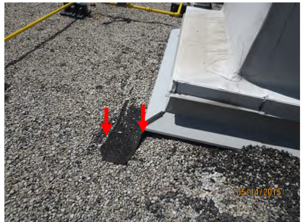
Photograph 20 – East view of Unit in Photo#19 Red arrow – open FR40 flashing lapstern
