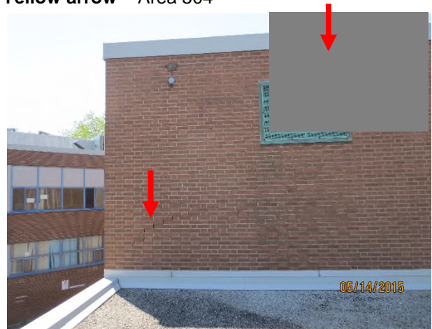
Photograph 4 – South-east corner on Area 303 (North-east wall of Area 502) Red arrow – cracked mortar joints and loose/dislodged bricks
