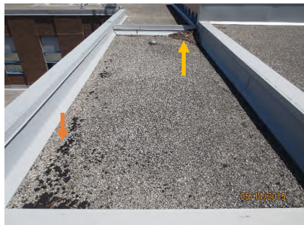
Photograph 30 – East view of Area 505 Yellow arrow – debris/vegetation Orange arrow – some asphalt bleed through – not a concern at this time
