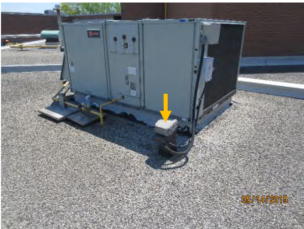
Photograph 7 – Close-up view of HVAC unit on Area 302 from Photo#6 Yellow arrow – conduit cap not secured
