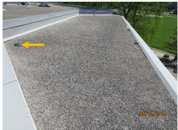
Photograph 18 – S/E view of area 401 Yellow arrow – damaged drain cover
