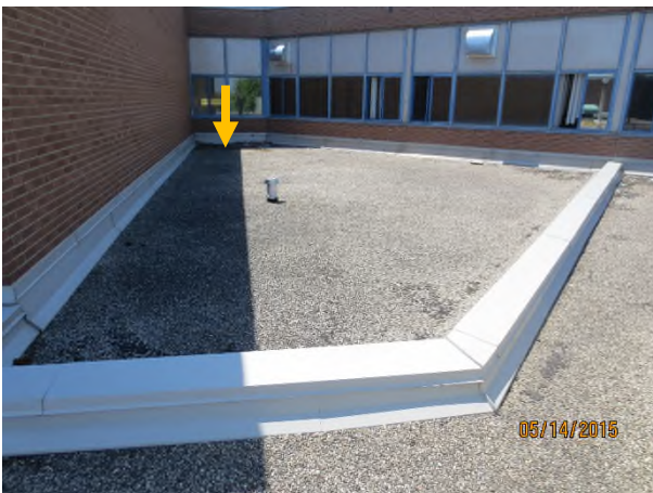
Photograph 5 – West view of Area 301 Yellow arrow – debris/vegetation on roof surface and around drain
