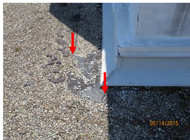
Photograph 12 – North side of Unit on Area 501 in Photo#9 Red arrow – open FR40 flashing laps
