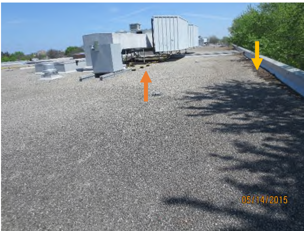
Photograph 19 – N/E view of Area 502 Yellow arrow – excessive vegetation growth along east wall (tree line) Orange arrow – vegetation growth under platform
