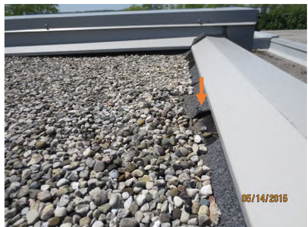
Photograph 34 – NW corner of Area 701 Orange arrow – mod. bit. cap sheet flashings in asphalt with some side laps open
