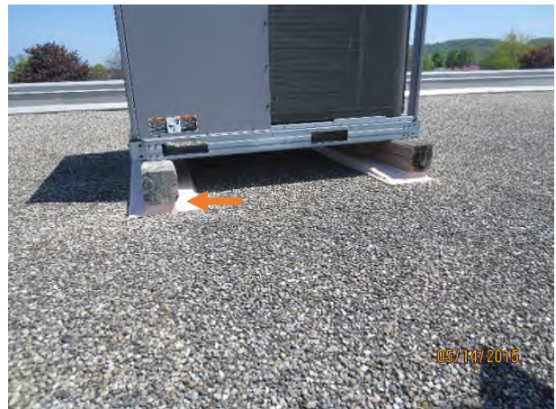
Photograph 32 – East view of A/C unit on Area 504, Photo#31 Orange arrow – deteriorated insulation under wood sleepers
