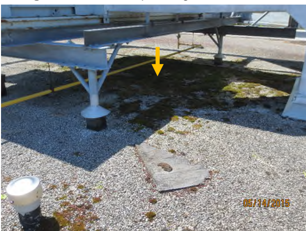
Photograph 11 – View of typical mechanical platform in Photo#9 Yellow arrow – vegetation/moss growth under platform
