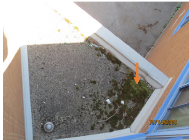
Photograph 38 – North view of Area 201 Orange arrow – moss growth on roof surface
