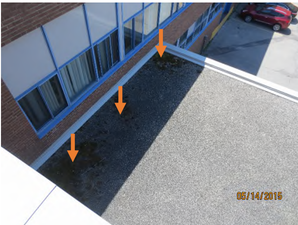
Photograph 25 – South side of Area 304 Orange arrows – debris/vegetation/moss growth
