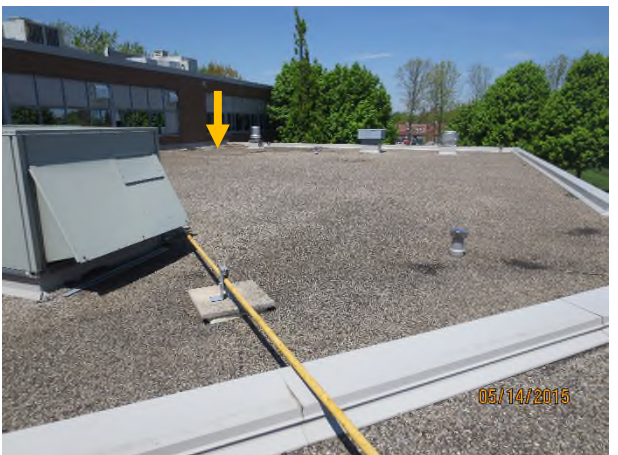
Photograph 6 – N/W view of Area 302 Yellow arrow – debris/vegetation on roof surface and around drains
