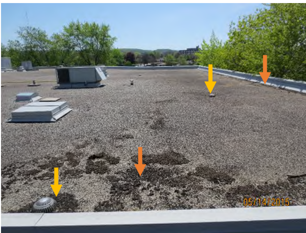
Photograph 15 – South view of Area 502 Yellow arrows – vegetation clogging drains Orange arrow – dry vegetation
