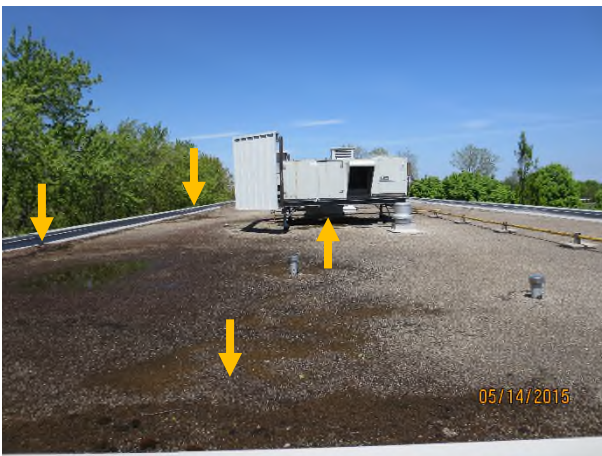
Photograph 9 – North view of Area 501 Yellow arrows – excessive vegetation growth along west wall (tree line) on roof area Orange arrow – water ponding
