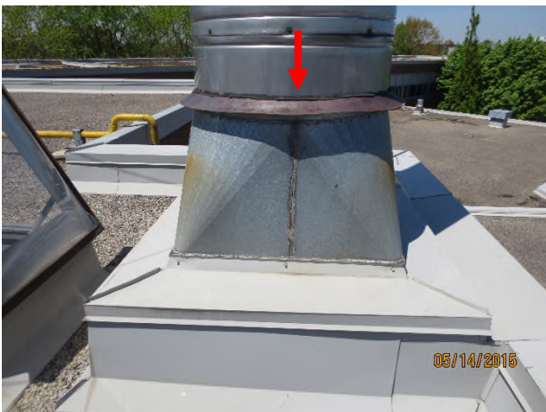
Photograph 17 – East side of stack in Area 502 Red arrow – cracked caulking
