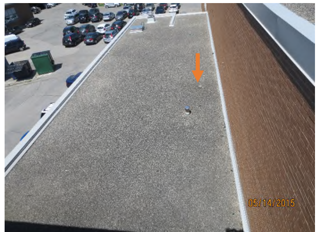
Photograph 24 – North view of Area 304 Orange arrow – debris/vegetation around drain
