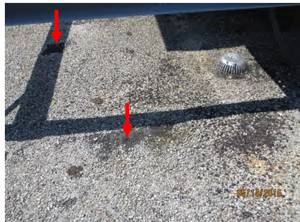
Photograph 10 – East view of Unit on Area 501 in Photo#9 Red arrows – exposed bitumen and felt
