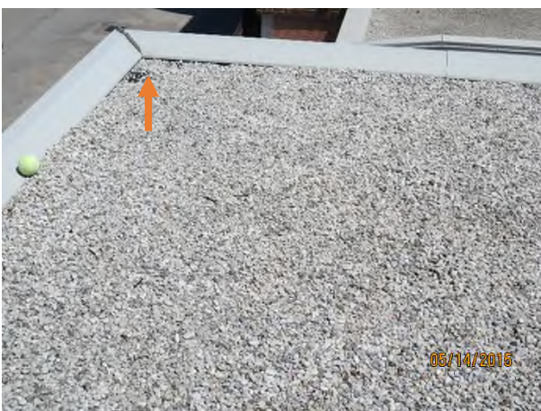
Photograph 40 – Example of wind scouring at N/E corner on Area 402
