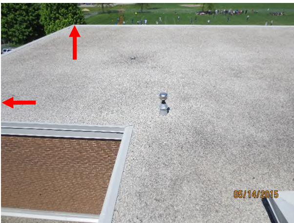
Photograph 27 – North view of Area 402 Red arrow – wind scouring at corners, otherwise roof surface in good condition and drains well
