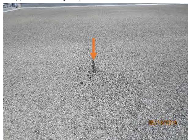
Photograph 41 – East view on Area 601 Orange arrow – membrane blister on roof surface
