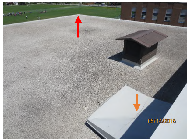
Photograph 28 – N/E view of Area 402 Red arrow – wind scouring at corner Orange arrow – damaged fan hood
