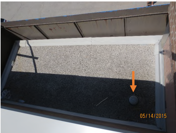
Photograph 37 – North view of Area 204 Orange arrow – minor debris around drain, roof in good condition
