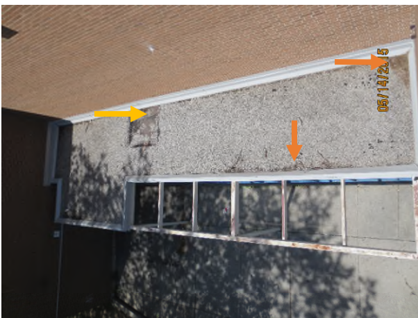
Photograph 39 – West view of Area 203 Orange arrow – minor debris/vegetation Yellow arrow – debris/vegetation at scupper
