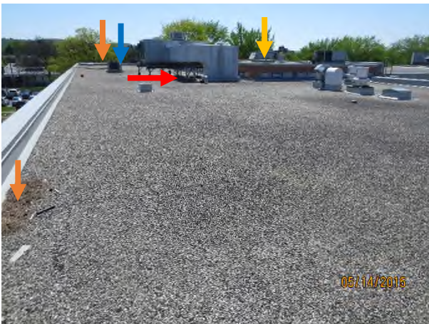
Photograph 31 – S/W view of Area 504 Orange arrows – debris/vegetation, Yellow arrow – Area 701, Red arrow – vegetation under mechanical platform, Blue arrow – insulation pad under A/C unit deteriorating
