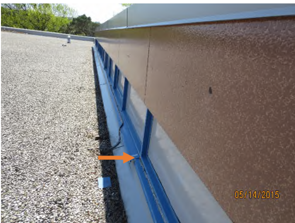
Photograph 35 – South view of east wall of Area 701 in Photo#33 Orange arrow – loose metal flashing at window sill, not weather tight below and failed sealant
