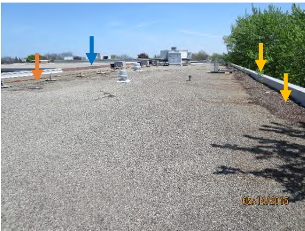
Photograph 21 – East view of Area 503 Yellow arrows – vegetation and tree growth Orange arrow – clogged drain Blue arrow – failed transition between Areas 601 and 503
