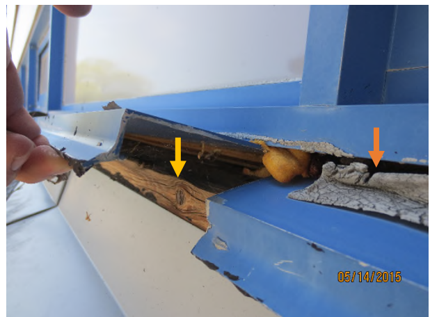
Photograph 36 – Close up view of window sill in Photo#35 Yellow arrow – no membrane flashing on wood Orange arrow – failed/cracked sealant
