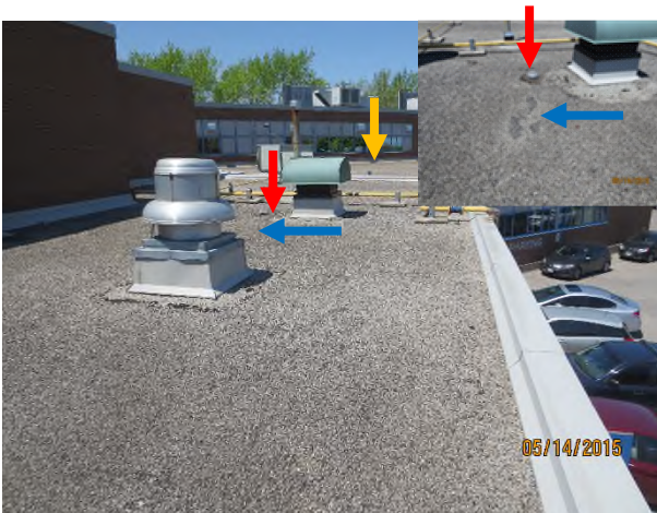
Photograph 3 – N/W view of Area 303 Red arrow – debris/vegetation on roof surface Blue arrow – membrane blister Yellow arrow – Area 302
