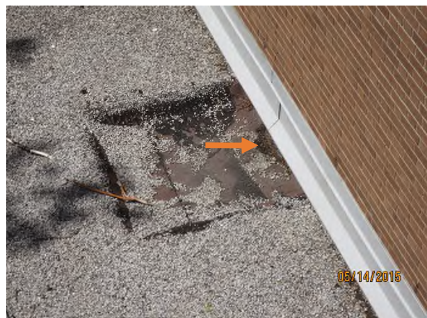
Photograph 40 – Close-up of depression/sump in Photo#39 Orange arrow – debris/vegetation clogging scupper, cleaning required
