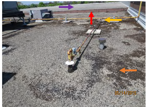
Photograph 22 – North view from Area 503 Orange arrow – dry vegetation, Yellow arrow – missing gas line support, Purple arrow – Area 601 Red arrow – cap sheet slippage, blistering, open laps at transition between 503 & 601
